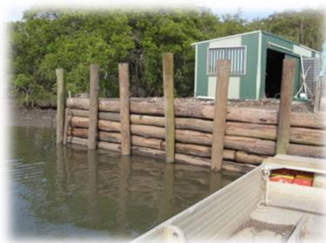
(R) Repairs made to retaining walls to improve erosion control.
