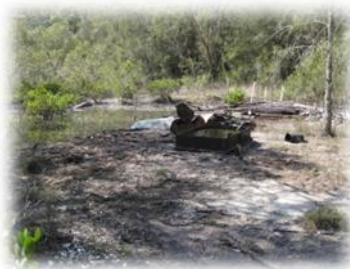
(Below) Removing 'old school' tar pots
