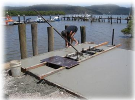
(L) Addressing erosion and suspended sediment input by constructing sediment traps.
