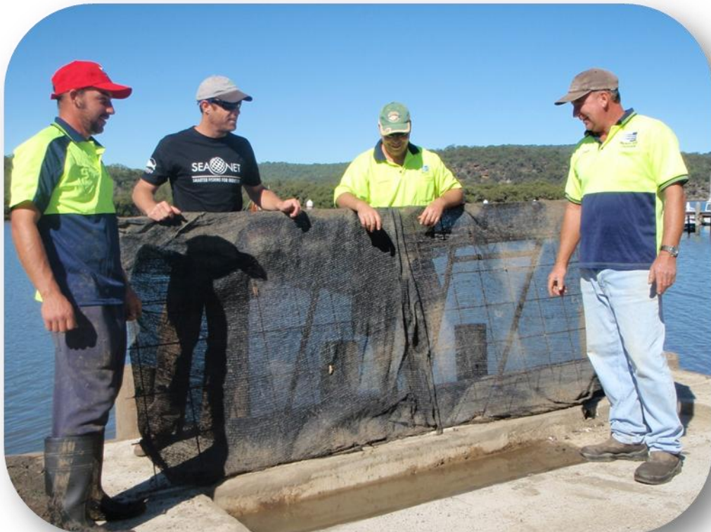
Figure 15. Inspecting the sediment control drains implemented at the land based facilities.
