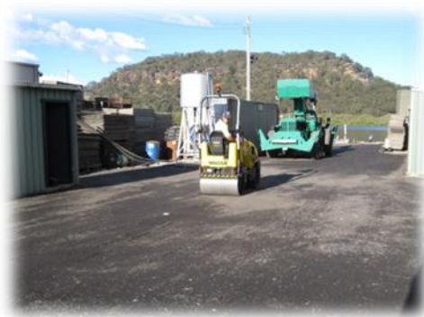
(R) Compacting and improving surface coverage to reduce dust and erosion.
